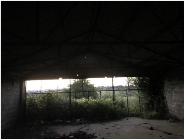
Plate 10: Internal view of derelict shed
