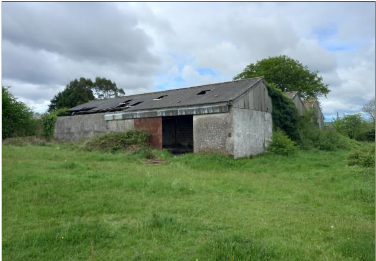
Plate 11.6: View of the 20 th century former industrial structures extant in Field 2
